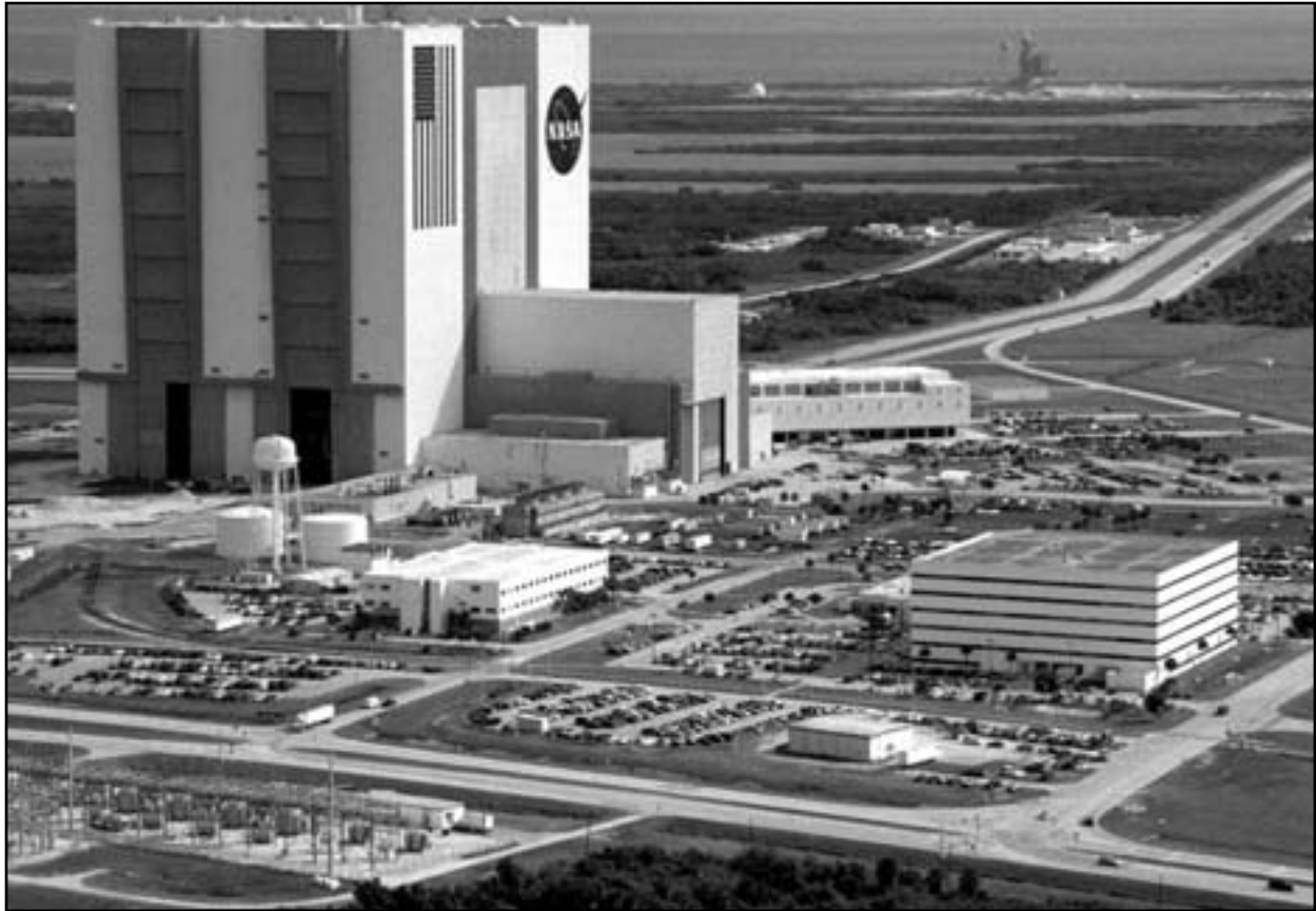
Figure 16. An aerial view of the Launch Complex 39 area shows the Vehicle Assembly Building (center), with the Launch Control Center on its right. On the west side (lower end) are (left to right) the Orbiter Processing Facility, Process Control Center, and Operations Support Building. To the east (upper end) are Launchpads 39A (right) and 39B (just above the VAB). The crawlerway stretches between the VAB and the launchpads toward the Atlantic Ocean, seen beyond them. (NASA Image 99PP-1213, also available at http://grin.hq.nasa.gov/ABSTRACTS/GPN-2000-000855.html )
