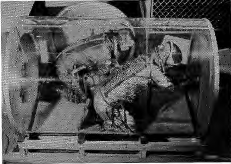
Two Langley engineers test an experimental air lock between an arriving spacecraft and a space station portal in January 1964.
