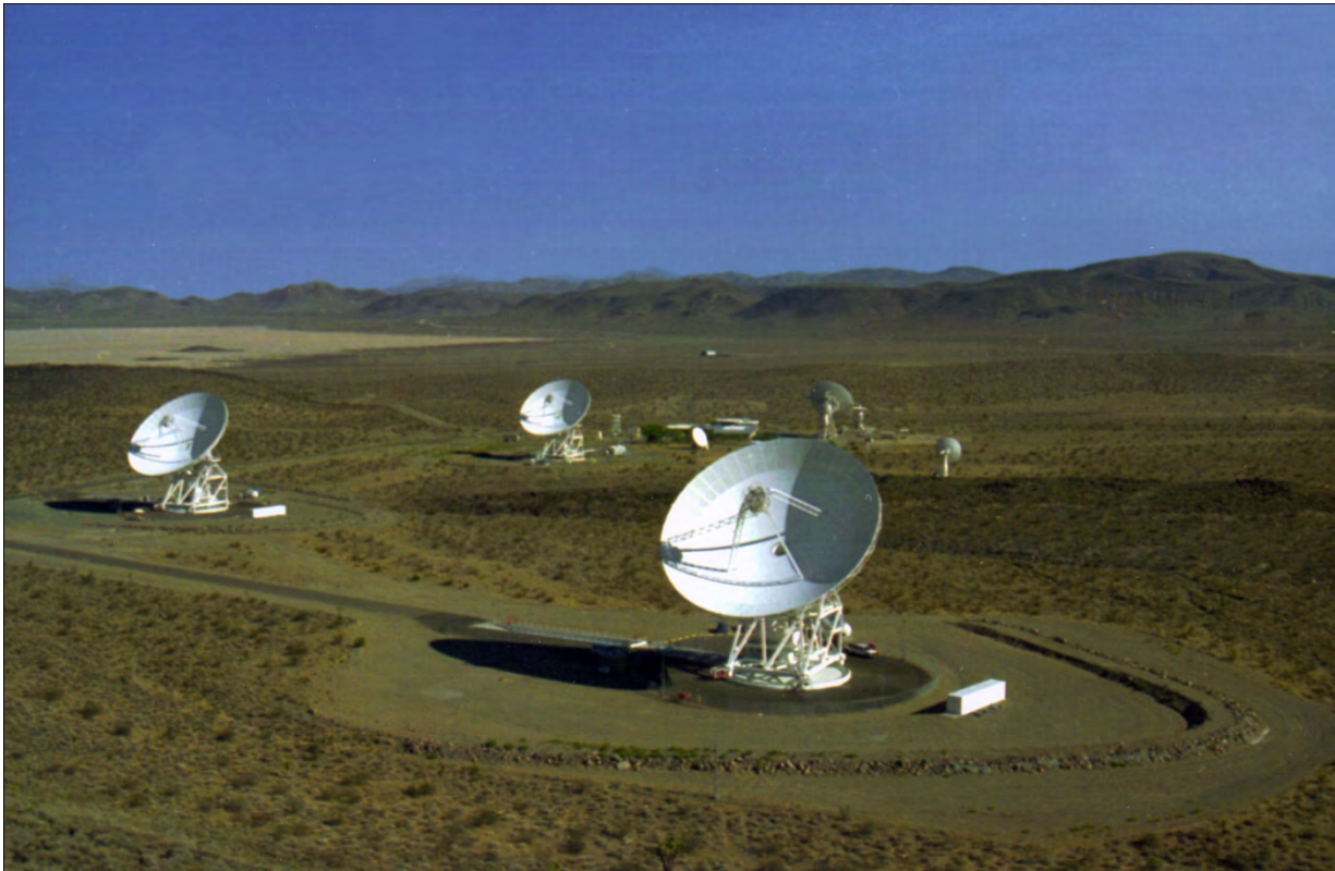
Figure 4-7. This photo shows three 34-meter (111-foot)-diameter beam waveguide antennas at the Goldstone Deep Space Communications Complex (NASA photo GPN-2000-000506).
