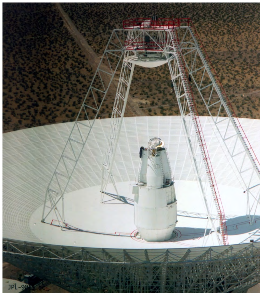
Figure 4-6. This photo shows the structure housing the electronics on the 70-meter (230-foot) antenna at the Goldstone Complex. Note the size of the person on the ladder at the center of the vertical pointing antenna in comparison to the size of the dish (NASA photo JPL 9015).
