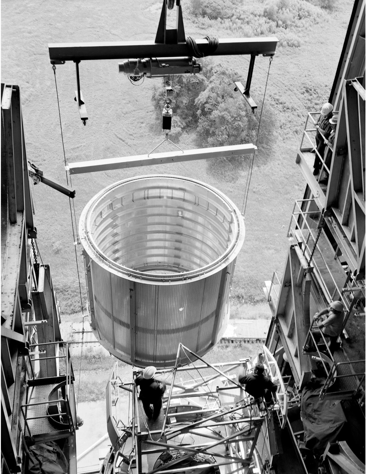
*Image 150: The Centaur D-1T's interstage adapter is lifted into the Nuclear Rocket Dynamics and Control Facility (B-3 Stand) during August 1972. The staff was preparing for upcoming Centaur Standard Shroud tests (GRC-1972-C-02855).*
