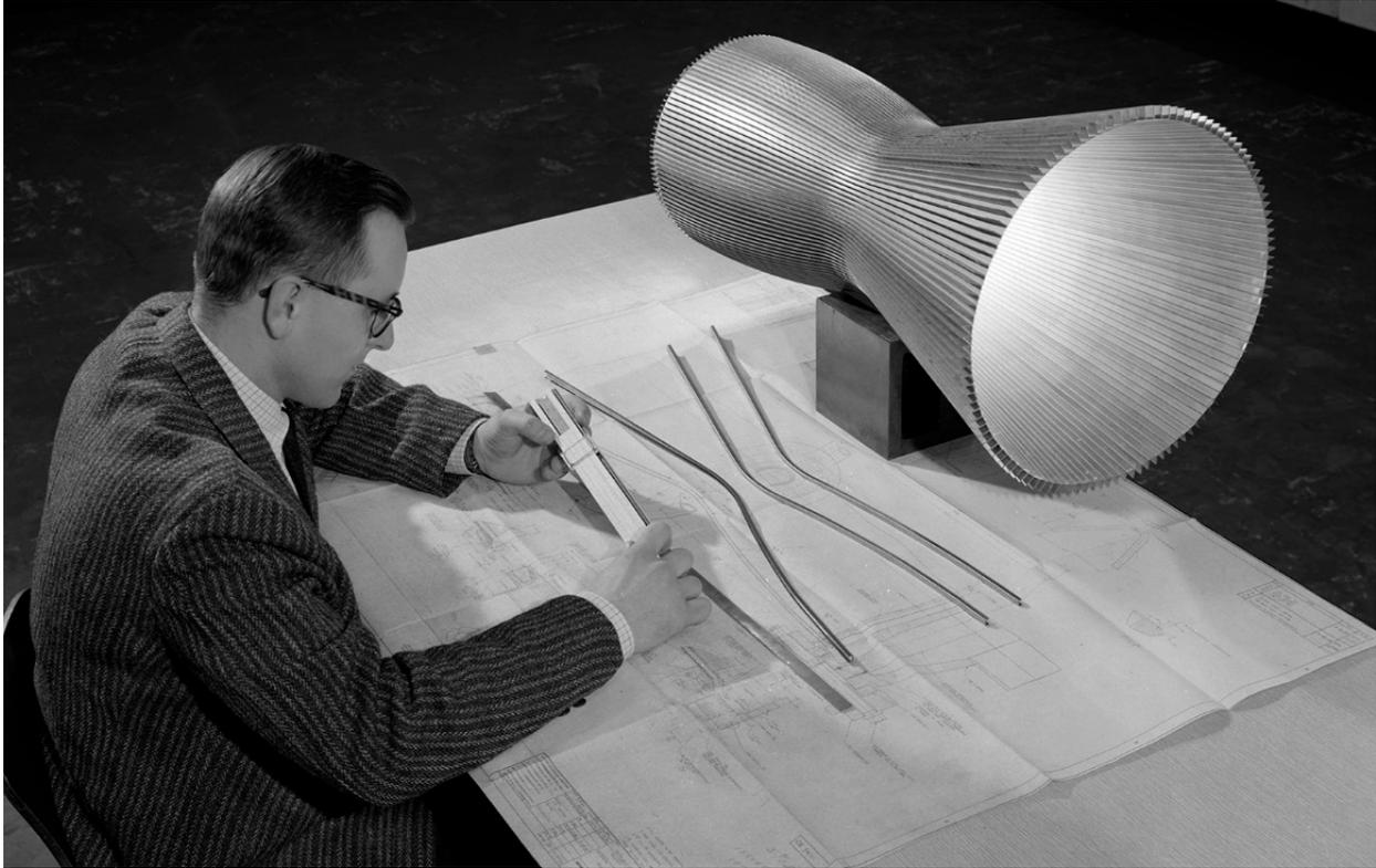
*Image 57: A Lewis engineer examines a drawing showing the assembly and details of a 20,000-pound-thrust regeneratively cooled rocket engine (GRC-1958-C-49377).*
