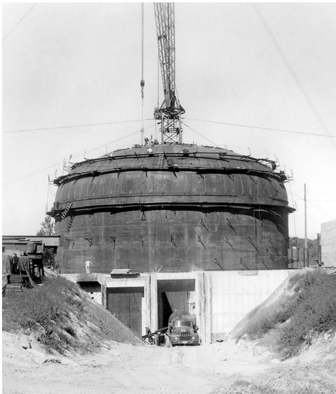
*Image 22: Construction of the reactor's containment vessel c1958. The reactor took five years to complete. By that time, most of the Rocket Systems Area sites were operational (GRC-2016-C-05109).*
