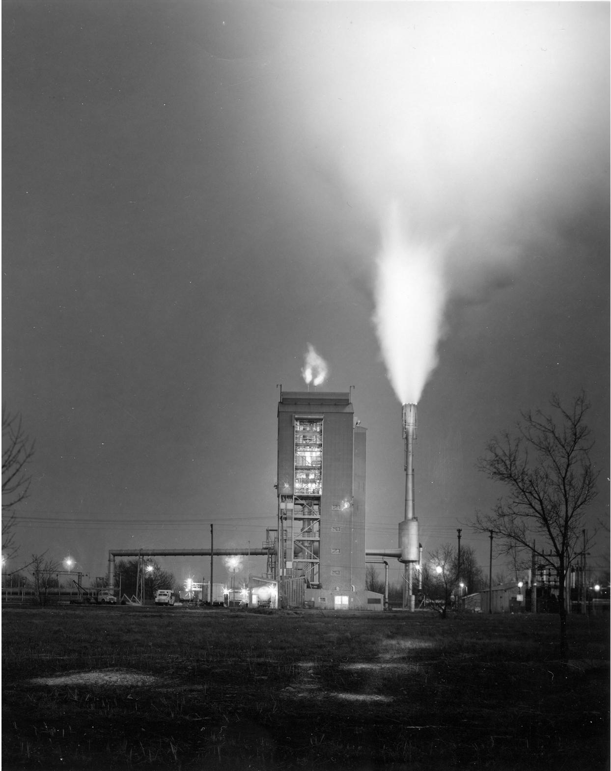
*Image 1: Testing of a hydrogen flow system for a nuclear engine in the High Energy Rocket Engine Research Facility (B-1 Stand) in June 1965 (GRC-1965-P-02327).*
