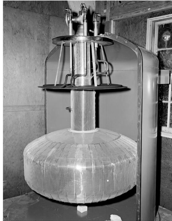
*Image 90: Insulated ADL calorimeter installation in the 5-foot-diameter J-3 test chamber (GRC-1963-P-01653).*
