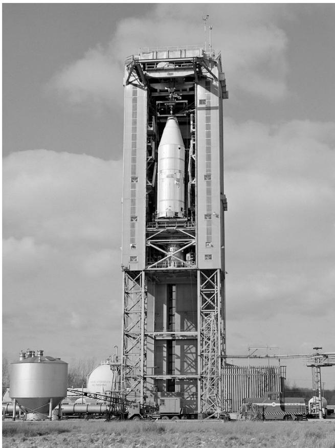
Image 164: CSS installed in the B-3 Stand (GRC-1973-C-01373).
