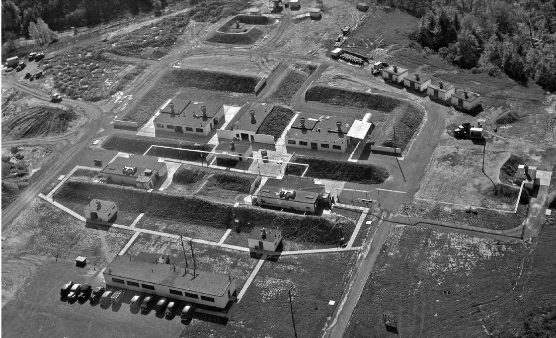
*Image 15: Rocket Lab shortly after Lewis's trades apprentices were enlisted to quickly construct protective earthen mounds around the facility in preparation for the 1949 Inspection (GRC-1949-C-24935).*
