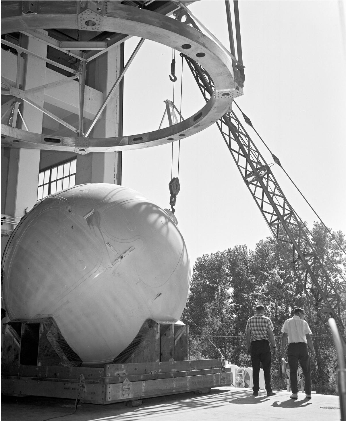
*Image 131: A 13-foot stainless steel tank is brought to K Site for pressurization tests in August 1966 (GRC-1966-P-01861).*
