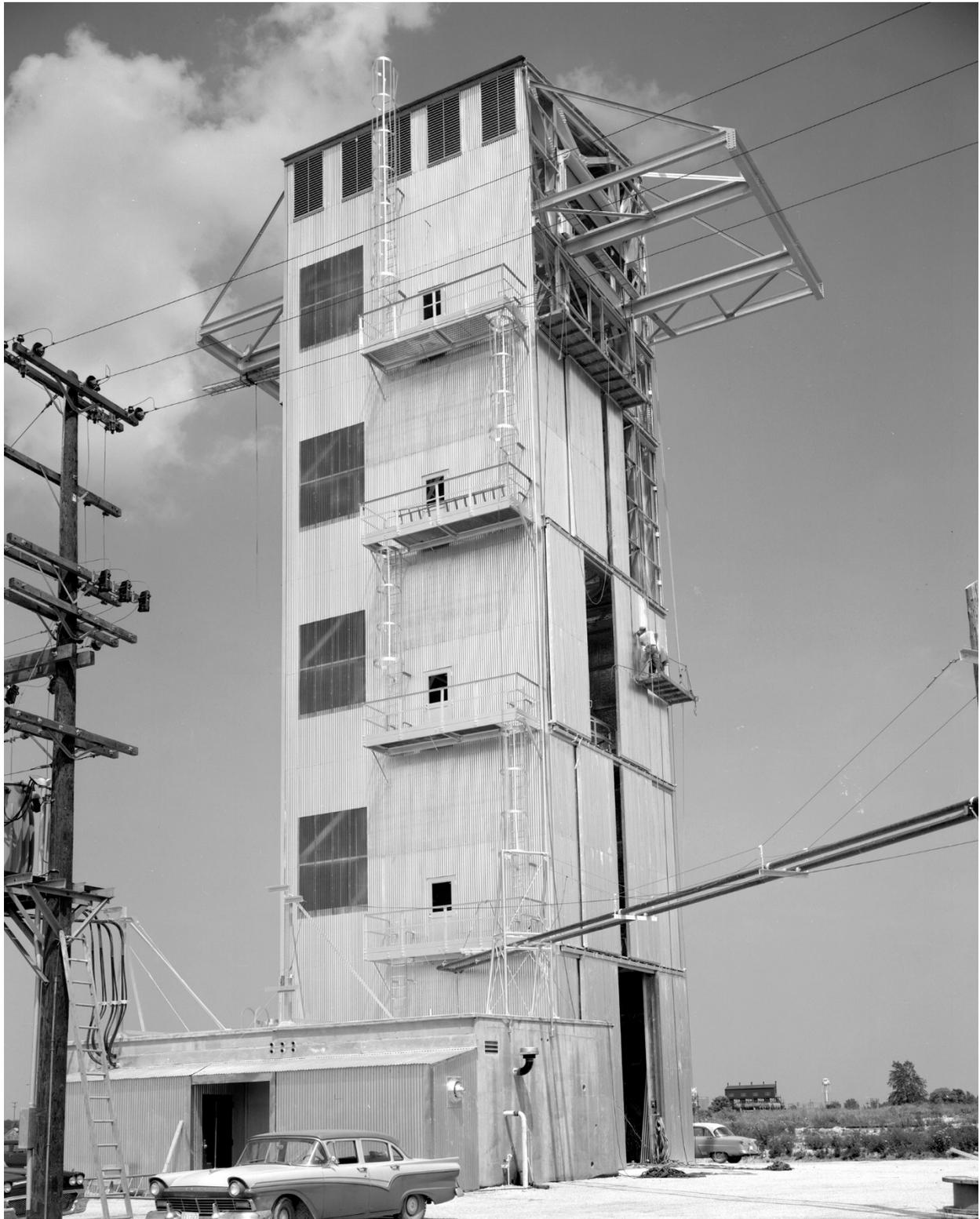
*Image 71: The Dynamics Stand as it nears completion in July 1959. The 144-foot-tall tower had a 14-foot-diameter well that ran the length of the structure to accommodate missiles (GRC-1959-C-51298).*
