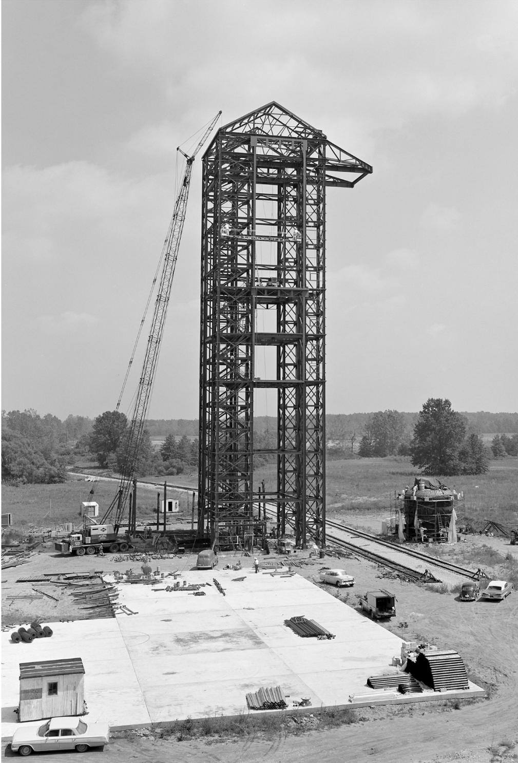
*Image 103: Construction of the B-3 Stand began in the spring of 1963.<sup>445</sup> Construction crews assembled the steel framework during the summer and added the siding and platforms in October. The basic structure was complete by mid-November 1963. The next year and a half were spent installing the other infrastructure and support systems, including the connection to the B-1 altitude exhaust system (GRC-1963-P-01751).*
