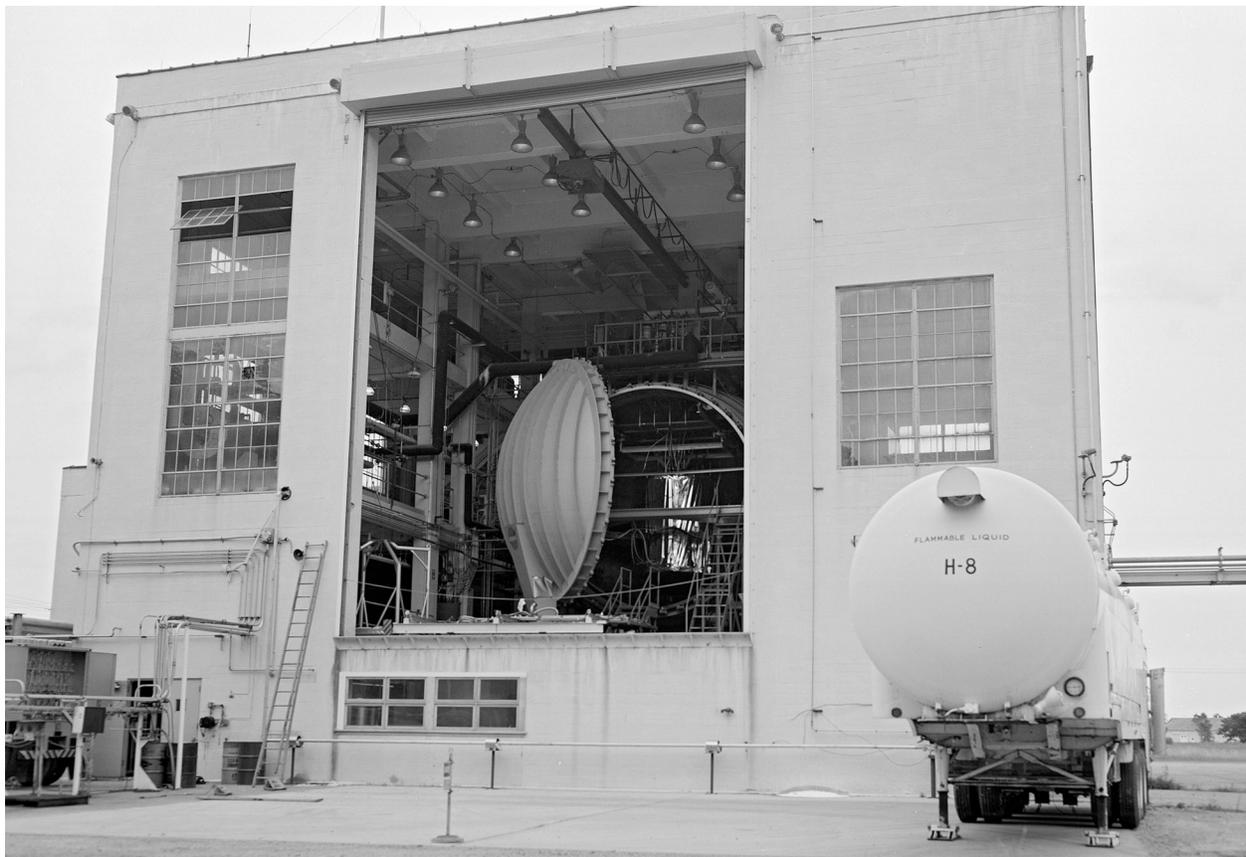
Image 147: K Site during the testing of the SEMI insulation. The cryoshroud is visible inside the test chamber (GRC-1971-P-1401).
