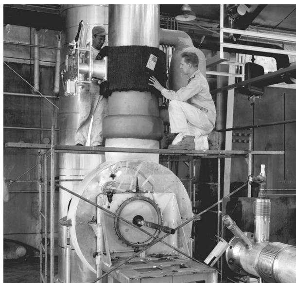
Image 187: Mechanic overhauls test loop at A Site (GRC-2016-C-05096).
