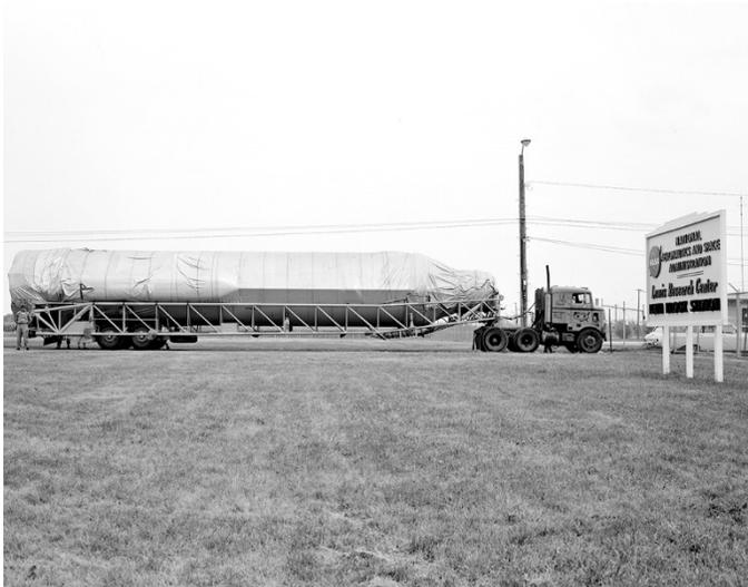
*Image 79: Atlas missile is delivered to Plum Brook in July 1963. The vehicle had to avoid tight turns, most bridges and underpasses, and large urban areas during its 2,500-mile trek from the General Dynamics plant in San Diego to Sandusky. (GRC-1963-C-65589).*
