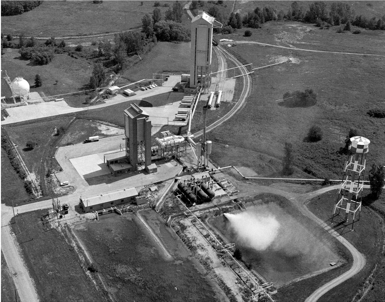
*Image 143: B-1 Stand firing in preparation for Centaur's pressurization system tests. Steam is emitted from the ejector of the facility's altitude exhaust system. The B-3 Stand is in the background (GRC-1966-C-04025).*
