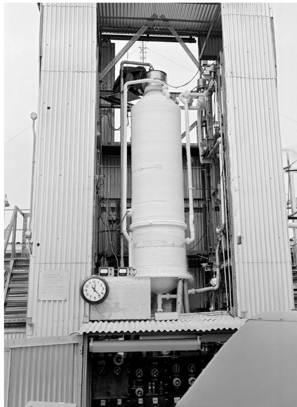
*Image 132: A tank is cold shocked with liquid nitrogen at J-4 during April 1962 (GRC-1962-C-01046).*
