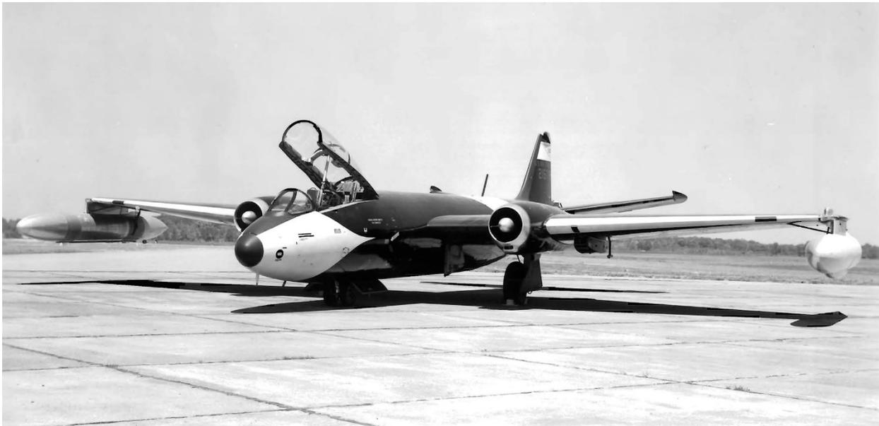
*Image 27: Martin B-57B Canberra used for Project Bee. The aircraft was powered by two Wright J65 engines—the one on the right was modified to operate on either jet fuel or liquid hydrogen. Lewis installed the two wingtip tanks. The one on the right stored the hydrogen and the one on the left contained the helium used to pressurize the flow system (GRC-2016-C-07419).*
