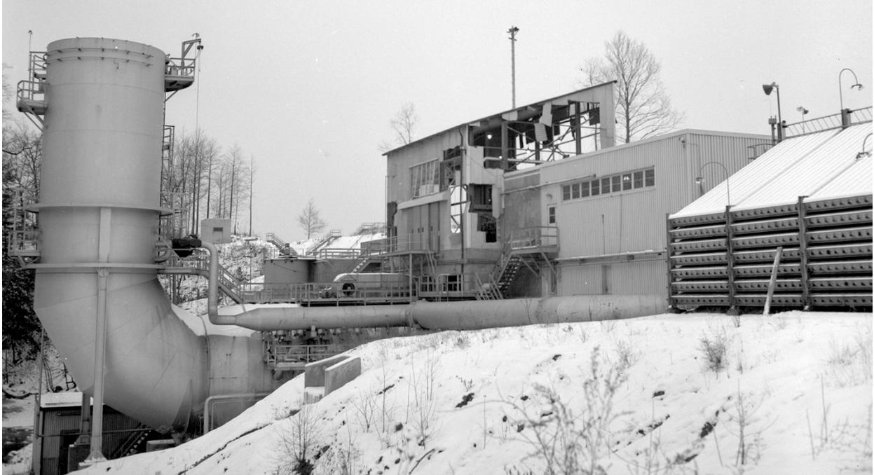
*Image 35: Damage to the RETF in December 1958. The RETF's first six months of operation were so eventful that Silverstein terminated fluorine testing at the site (GRC-1958-C-49372).<sup>175</sup>*
