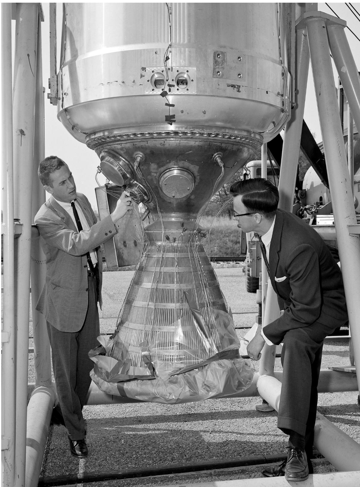
*Image 100: Researchers analyze a Kiwi B-1 engine before installation in the Nuclear Rocket Dynamics and Control Facility (B-3 Stand) in May 1967 (GRC-1967-P-01290).*
