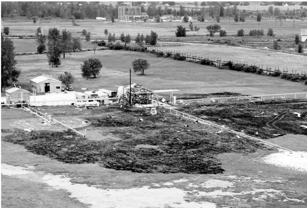
*Image 93: Damage at the Pilot Plant following a liquid-hydrogen explosion on 14 September 1964. The blast convinced engineers to install a protective concrete wall inside the H Control entrance (GRC-1964-P-1559).*
