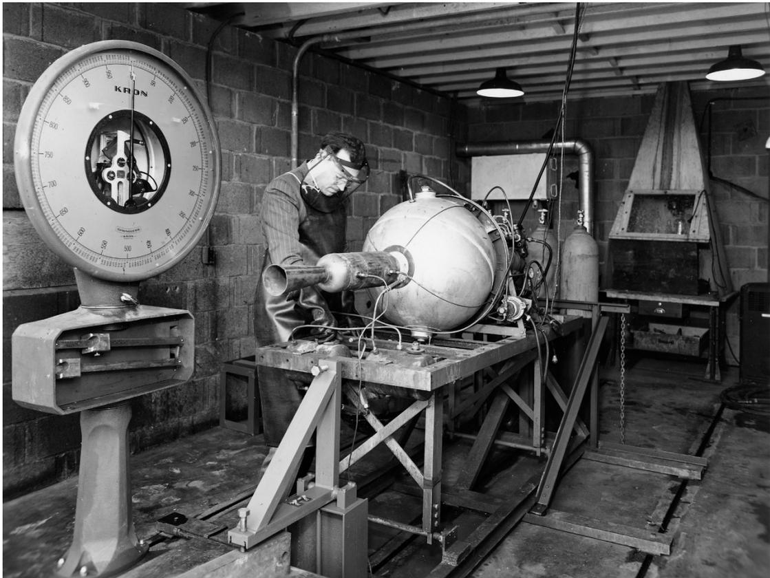
*Image 16: A Rocket Section researcher prepares a rocket engine for testing at the Rocket Lab with the hypergolic combination of nitric acid and aniline in March 1946 (GRC-1946-C-14482).*
