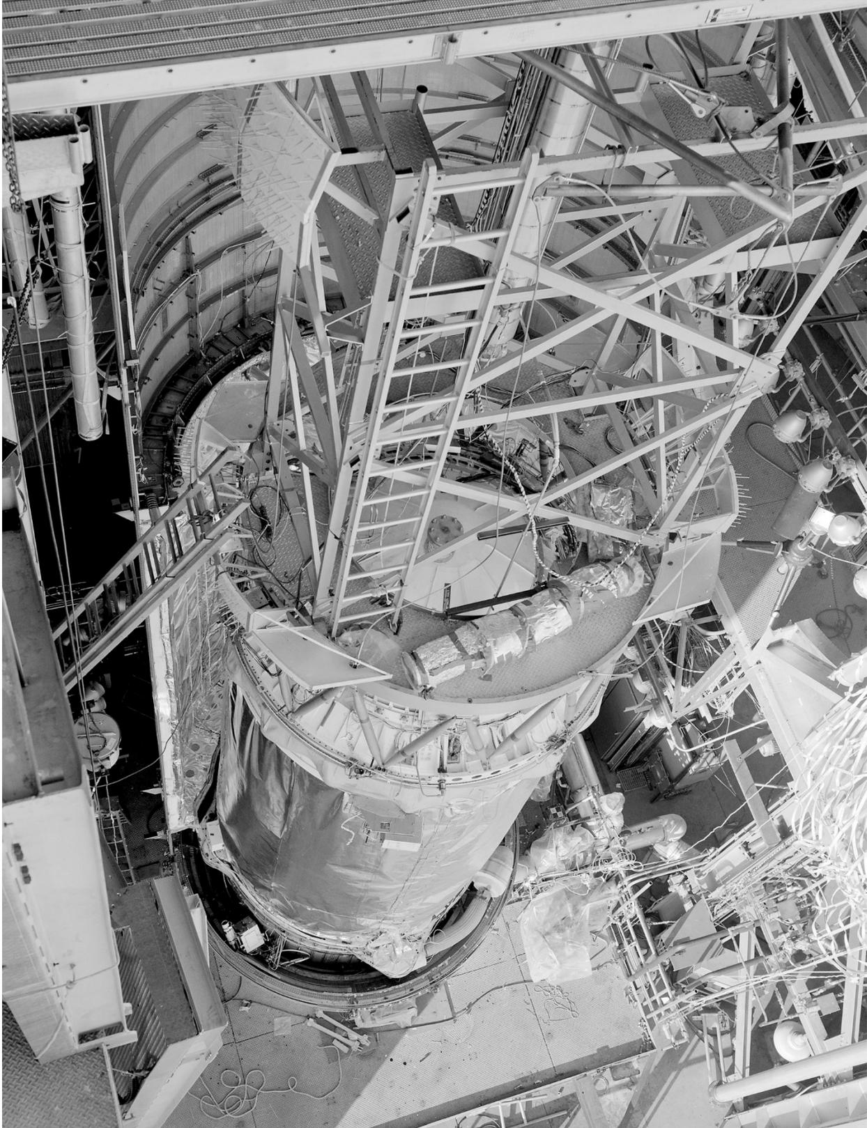
*Image 163: Preparations at the B-3 Stand for the structural test of the CSS in early 1973. The test setup included the Centaur, its interstage adapter, a flight-weight propellant tank, and a Viking model (GRC-1973-P-01383).*
