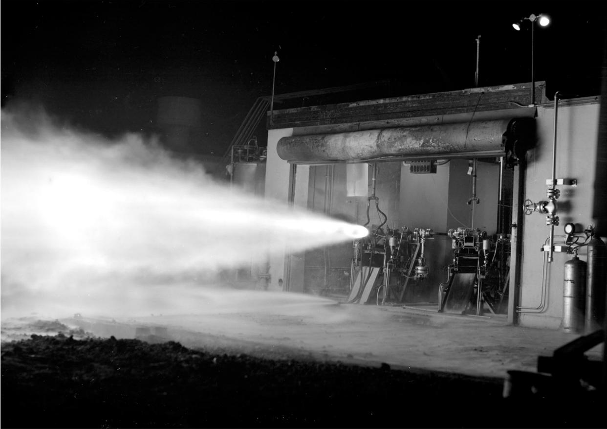
*Image 25: Firing of a 5,000-pound-thrust liquid-hydrogen/liquid-oxygen engine from Cell 22 of the Rocket Lab in early January 1955. It was part of Lewis's first series of hydrogen-oxygen engine tests, which were suspended to redesign the injector and engine controls (GRC-1955-C-37428).*
