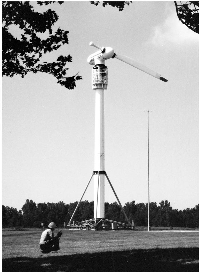
*Image 172: Single-bladed rotor. One of the most successful configurations used a lone blade with a counterweight on the other side. Despite concerns about the evenness and level of its power output, the single-bladed wind turbine generated over 200 kilowatts of power, twice the facility's original design capacity<sup>740</sup> (GRC-1985-C-05882).*
