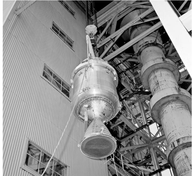
Image 192: Kiwi-B reactor is lifted into the B-1 Stand (GRC-1963-P-01358)
