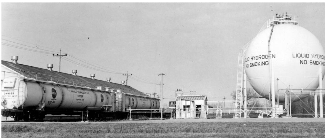
*Image 63: The 200,000-gallon liquid-hydrogen Dewar at B Complex. The container consisted of a thick steel shell that was protected by a 9-inch-thick multilayer foil-and-glass-wool insulation and was encapsulated by a thin outer shell (GRC–1965–P–02580).*
