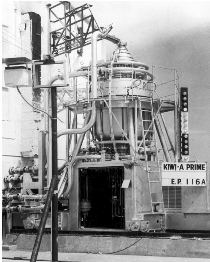
Image 40: Kiwi-A reactor preparations for test at Los Alamos (NASA CC-214).
