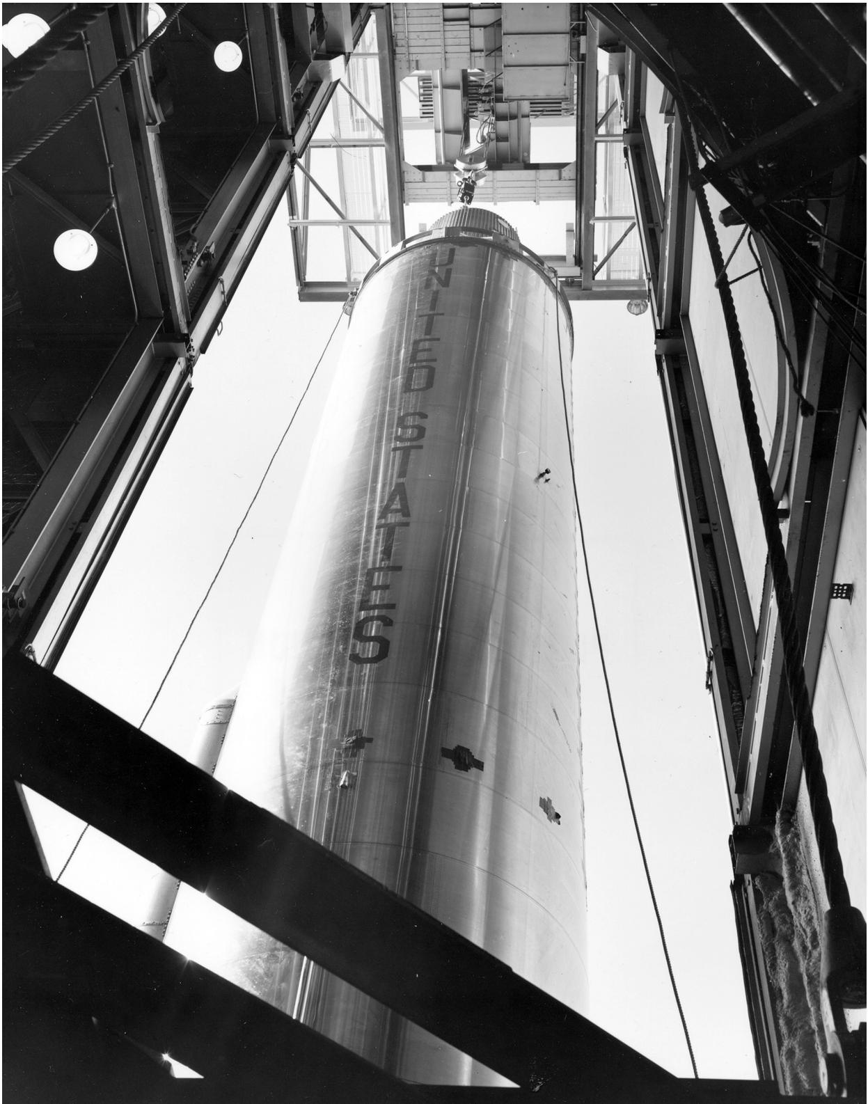
*Image 81: Installation of Atlas stage into E Stand in August 1963. The vehicle had to be pressurized during the process to avoid damage to the aluminum shell (GRC-1963-P-01716).*
