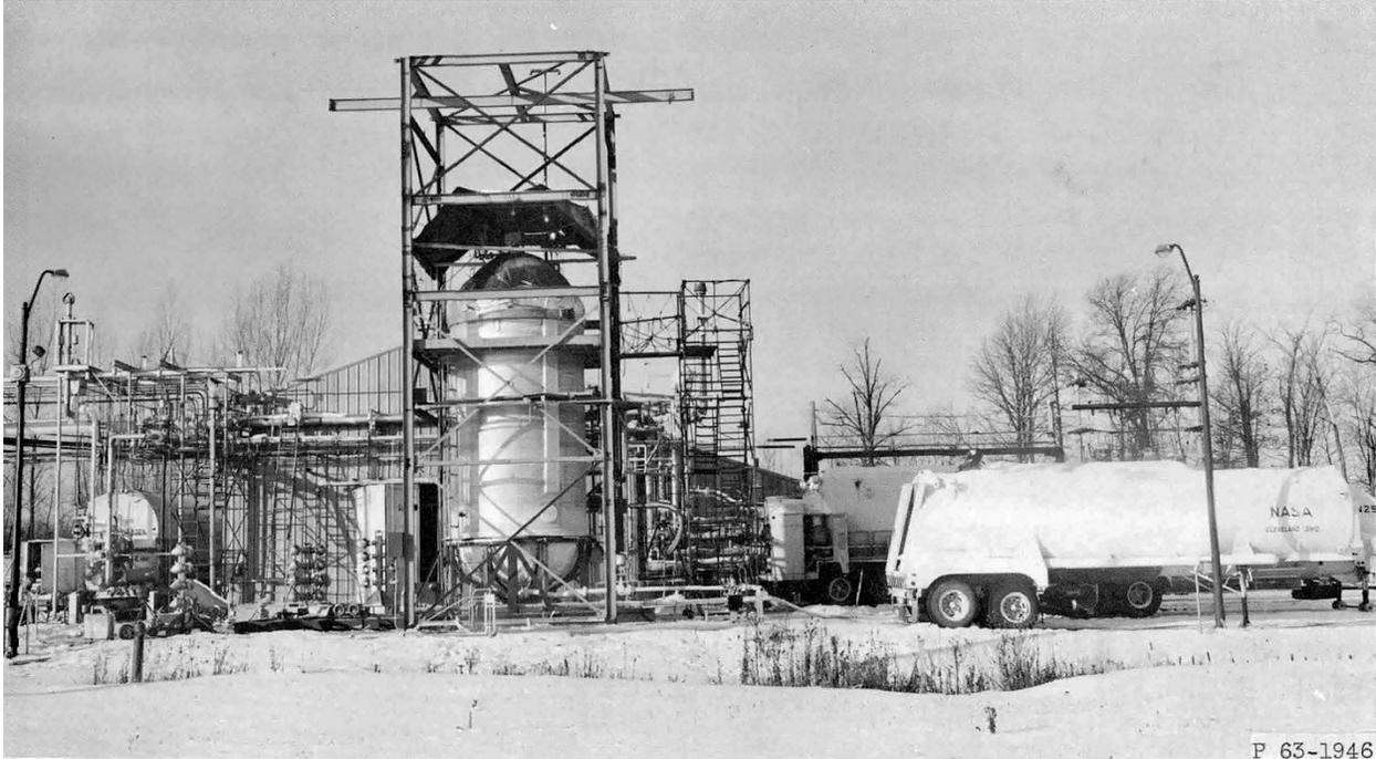
Image 78: Constrictively wrapped full-scale Centaur tank in the J-4 test stand. Twenty foam panels were affixed to the tank, covered with the Mylar and aluminum laminate, an aerodynamic shield, and the constrictive wrap (NASA TM X-52004, Fig. 10).
