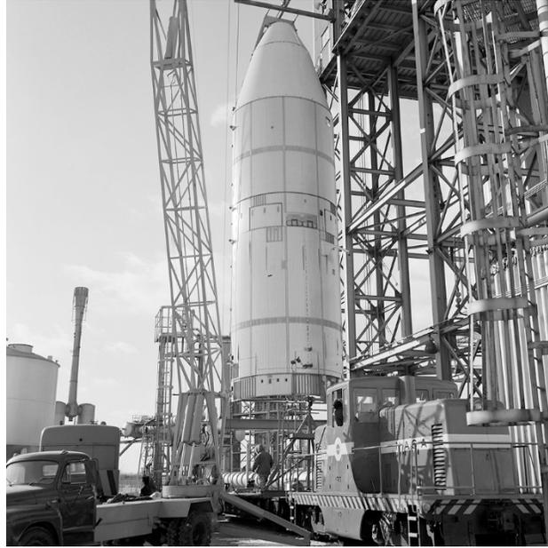
Image 196: CSS being loaded into the B-3 Stand (GRC-1973-P-01377).
