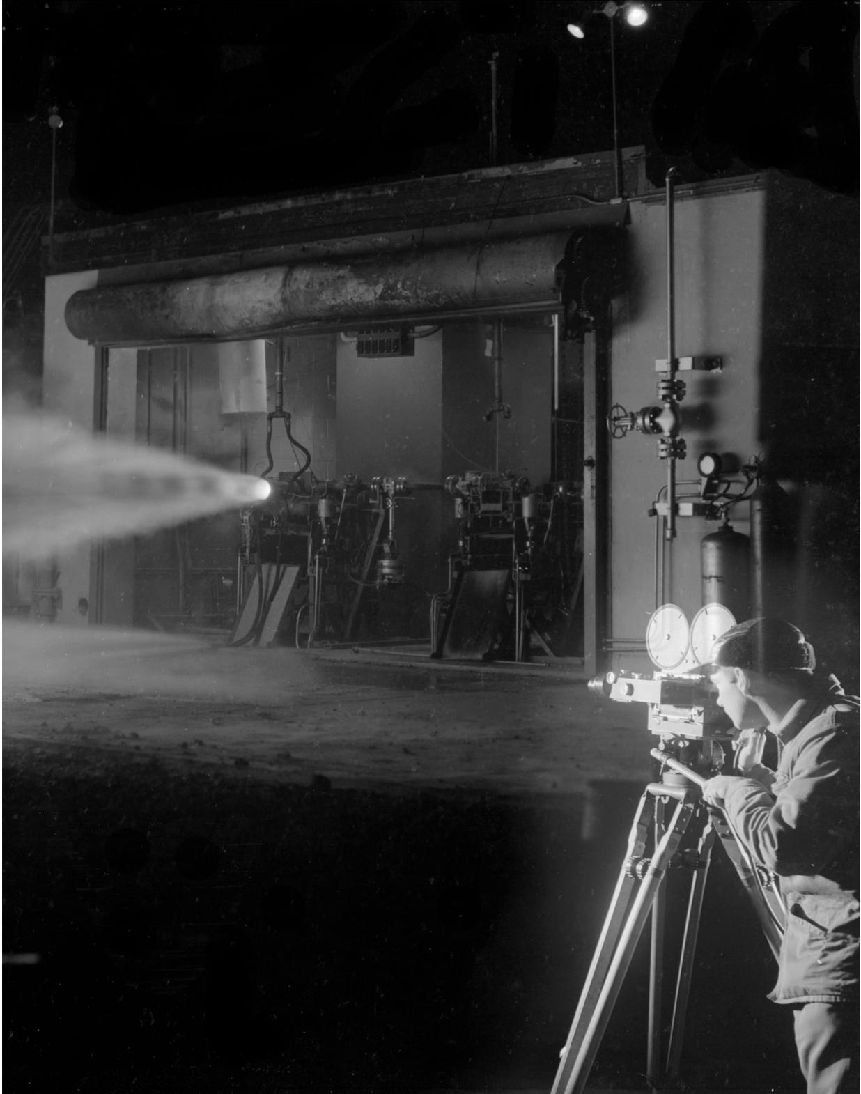
*Image 19: A Lewis photographer films the test of a liquid-hydrogen/liquid-oxygen engine in Cell 22 of the Rocket Lab during January 1955. Researchers used the film footage to analyze the combustion (GRC-1955-C-37427).*
