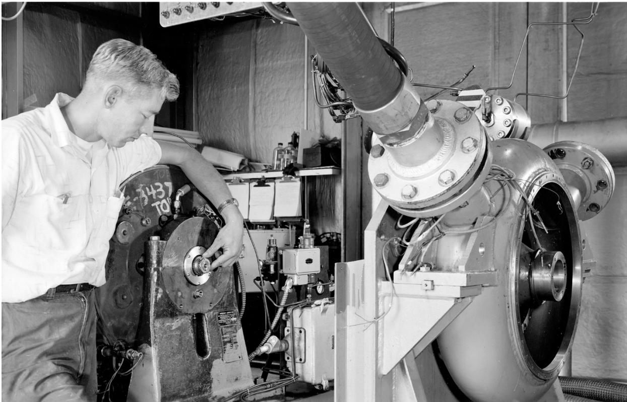
Image 45: Technician adjusting the setup of a gaseous-hydrogen turbine at the Pilot Plant in August 1960 (GRC-2016-C-05133).
