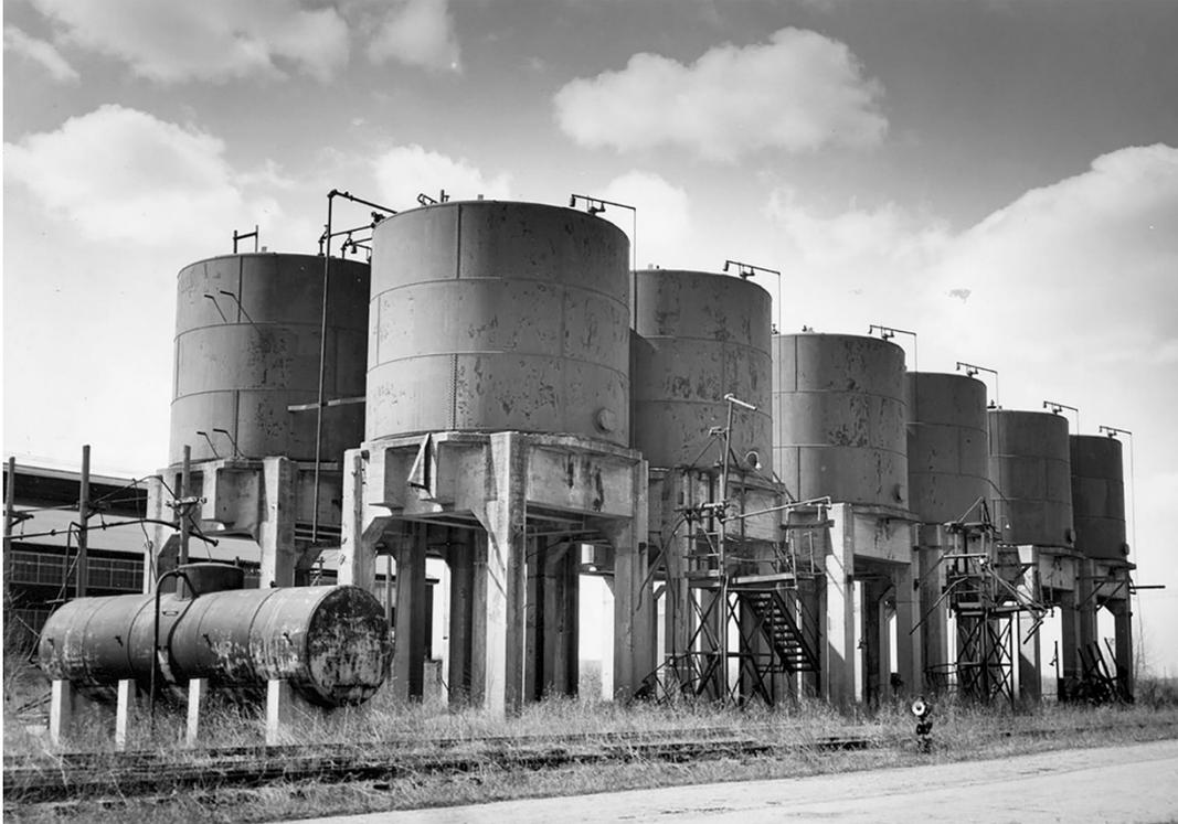
*Image 11: An Acid Area at the PBOW. The acid was used to manufacture TNT and DNT. The waxlike chemicals were scraped into flakes and stored in the PBOW's concrete bunkers until shipment to the Ravenna Arsenal for incorporation into shells (GRC-2016-C-05097).*
