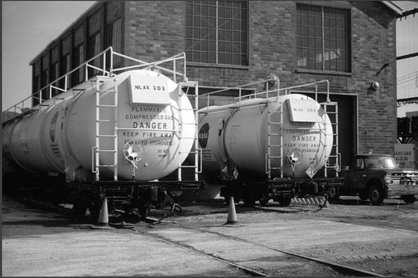
Image 64: Lewis’s railcar Dewars parked beside the Locomotive Shop at Plum Brook. The four railcars were later transferred to Cape Kennedy for the space shuttle program (GRC-2016-C-05187).
