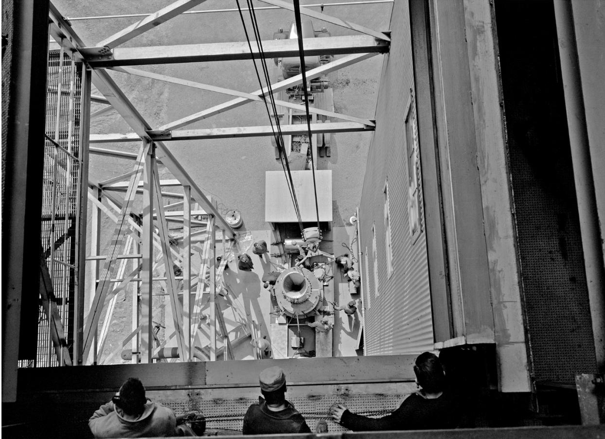
*Image 107: A Kiwi-B engine is hoisted into the B-1 Stand on 11 April 1963. After undergoing initial checkout runs, the engine was lowered for analysis of the reactor and its fuel elements. Issues with the new facility delayed the reinstallation and checkout work into January 1964 (GRC-1963-P-01355).*
