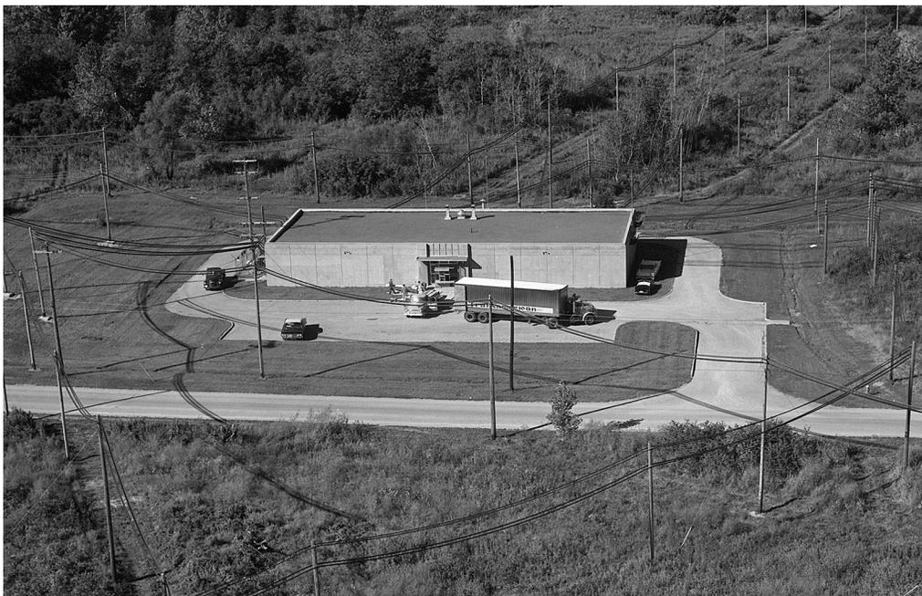
*Image 66: Control and Data Building (H Control Building), as seen in 1960, with its myriad of wires running out to the test sites. Universal Marine Construction Company was responsible for laying the 600 control cables, 500 pairs of instrumentation cables, and eight television lines emanating from these facilities in 1959.<sup>287</sup> The number of cables soon increased (GRC-1960-C-54934).*
