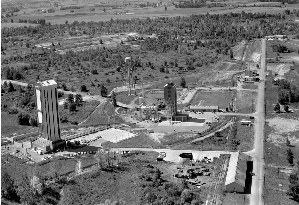
*Image 104: The B Complex included the Pump and Shop Building, a substation, two boiler buildings, a Valve House, and the steam ejector apparatus. The B Control Building is visible in the upper right corner (GRC-1964-C-72620).*
