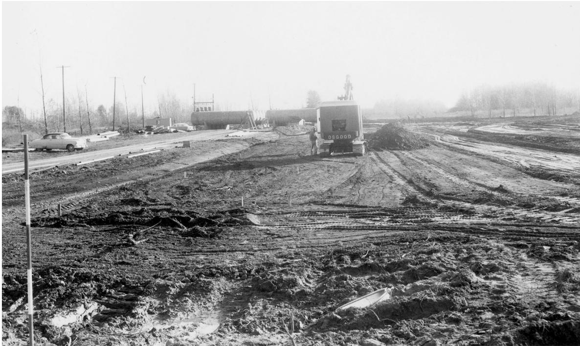
*Image 43: Grading and early construction work in the fall of 1958 at the Liquid Hydrogen Pump Facility (A Site). The facility's structures were in place in the spring of 1959. A Site began operations in 1961 (GRC-2016-C-05092).*
