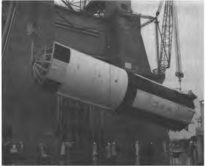
Installing S-IC-T stage in S-IC Test Stand in March 1965.
