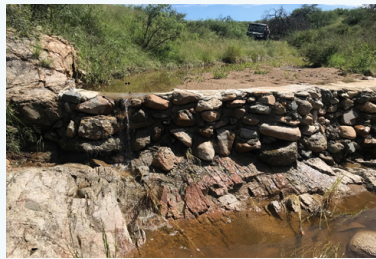
Examples of Natural Infrastructure in Dryland Streams (NIDS), including a) check dams at El Coronado Ranch; b) leaky weir at Cienega Ranch; and c) Zuni Bowl (One-rock Dam) at Cebolla Wilderness Area within the El Malpais National Conservation Area. Source: USGS.
