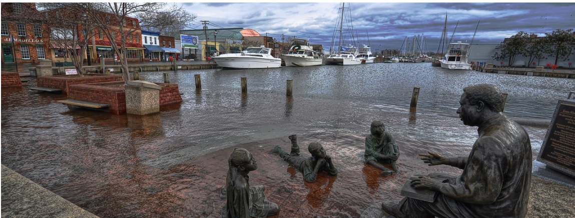
Annapolis, Maryland, affected by tidal flooding. Tidal flooding has increased dramatically across U.S. coastlines over the past 50 years as global average sea level has risen, driven by human-caused climate change. Credit: NOAA.
