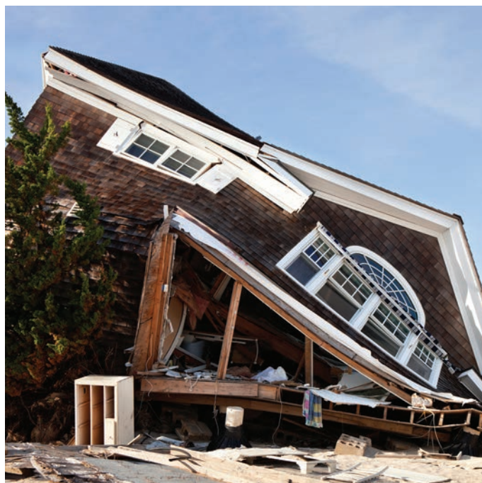
Storm-damaged home after Hurricane Sandy.
