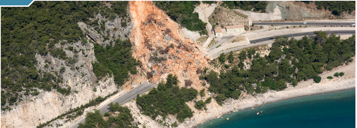
Landslide blocking a road in California
