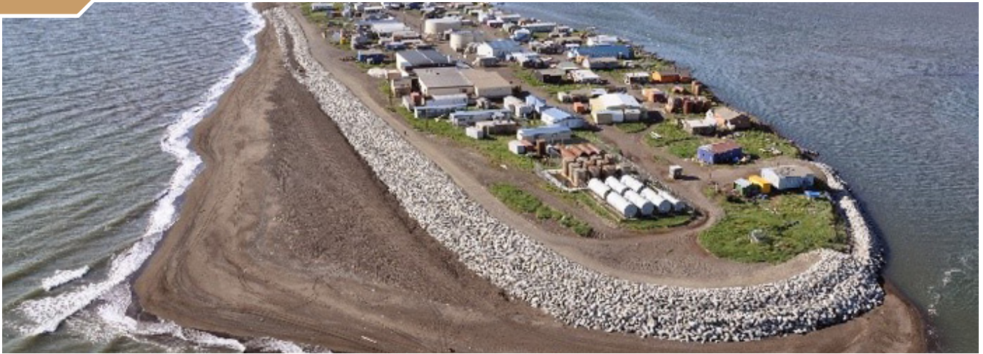
Seawall surrounding Kivalina, Alaska
