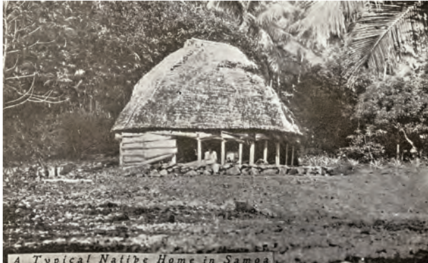
Figure 2. An early 20th-century photograph of a fale, a thatched pavilion without walls.
