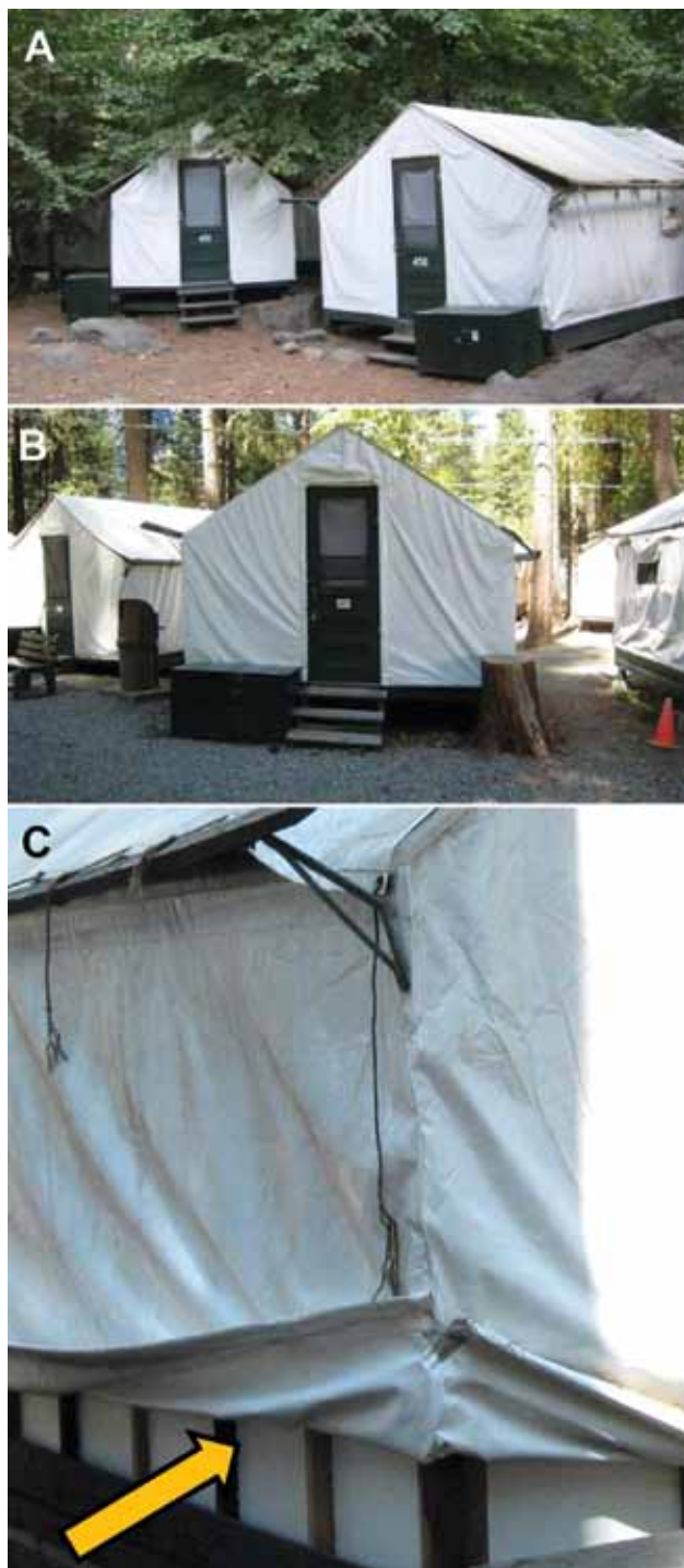
Figure 2. Regular and signature tent cabins, Yosemite National Park, summer, 2012. A) Outside view of a regular tent cabin. B). Outside view of a signature tent cabin. C) Inner layer of foam insulation under the canvas of a signature tent cabin.
